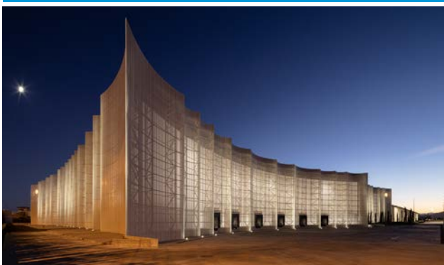
Total Clima Málaga - Logistic Center
