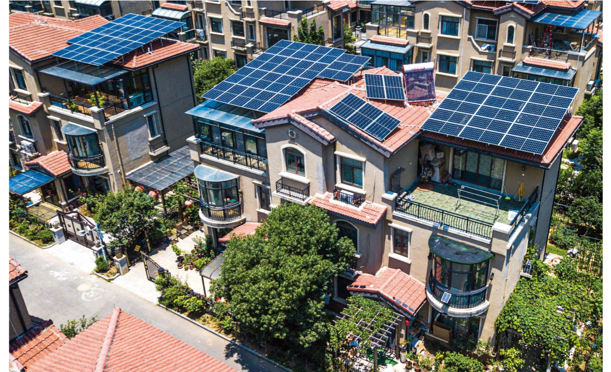
🏠 Anhui Chuzhou Villa Home PV Power Station Project
