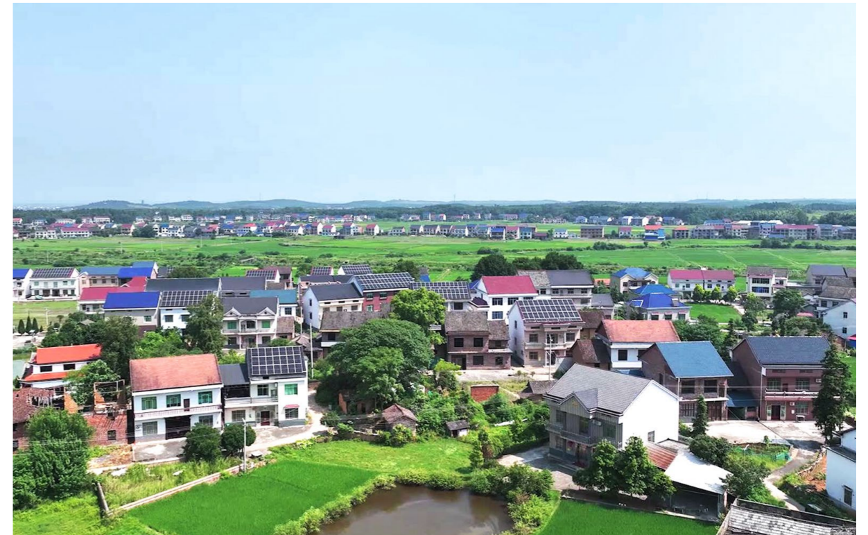
🏠 Hunan Youxian Residential Building PV Power Station Project
