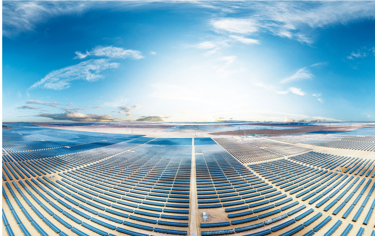
China's First Ultra-Large Grid-Parity PV Leader Project - Qinghai Geermu 500MW Power Station Project
