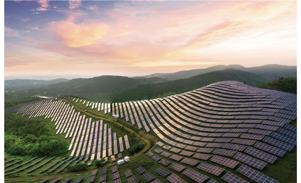
Anhui Chaohu 50MW PV Power Station Project
